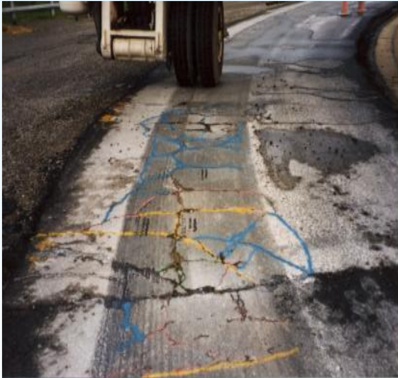
Fatigue experiment on asphalt pavement
