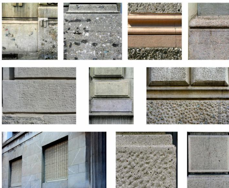
Fig. 1. Different kinds of imitation of stone (conglomerate, red or brown limestone, pink or white granite, veined marble etc.) executed using mortars made of Portland cement mixed with sands or crushed stones (early 20 th century, Milano, Italy)
