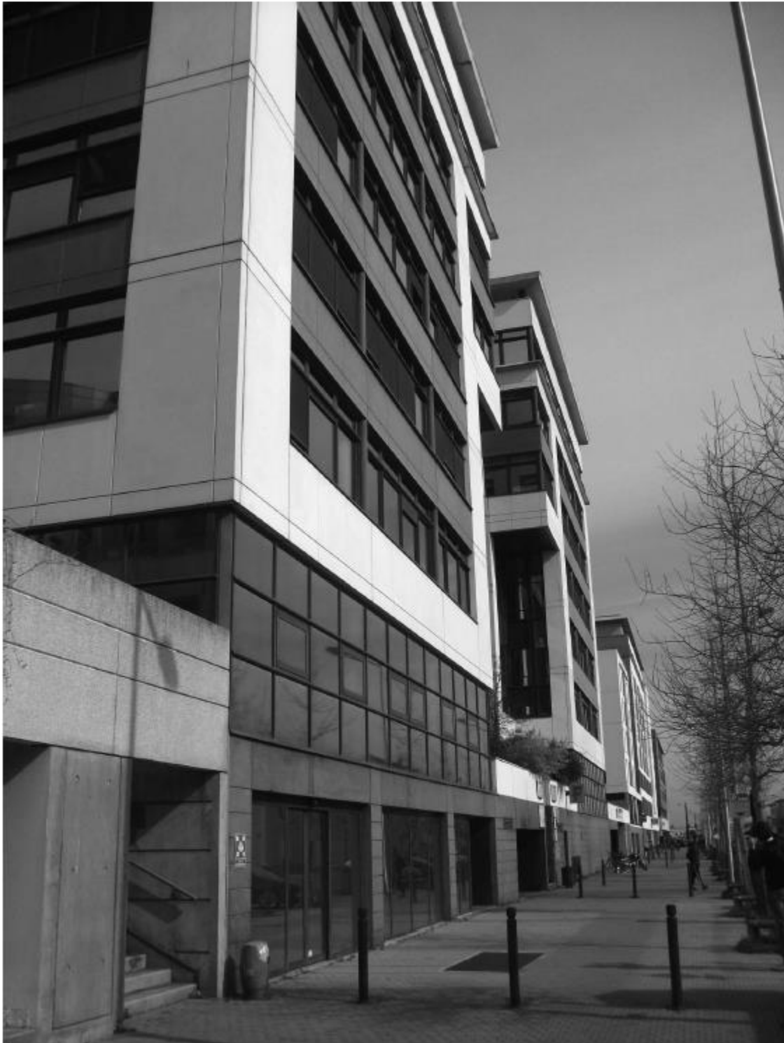
Figure 2 Example of an entrance to groundfloor parking and treatment of façades on the street side. Access for vehicles in the car park via a ramp. This device protects the car park and the first floor in case of flooding. Source: A. Moreau
