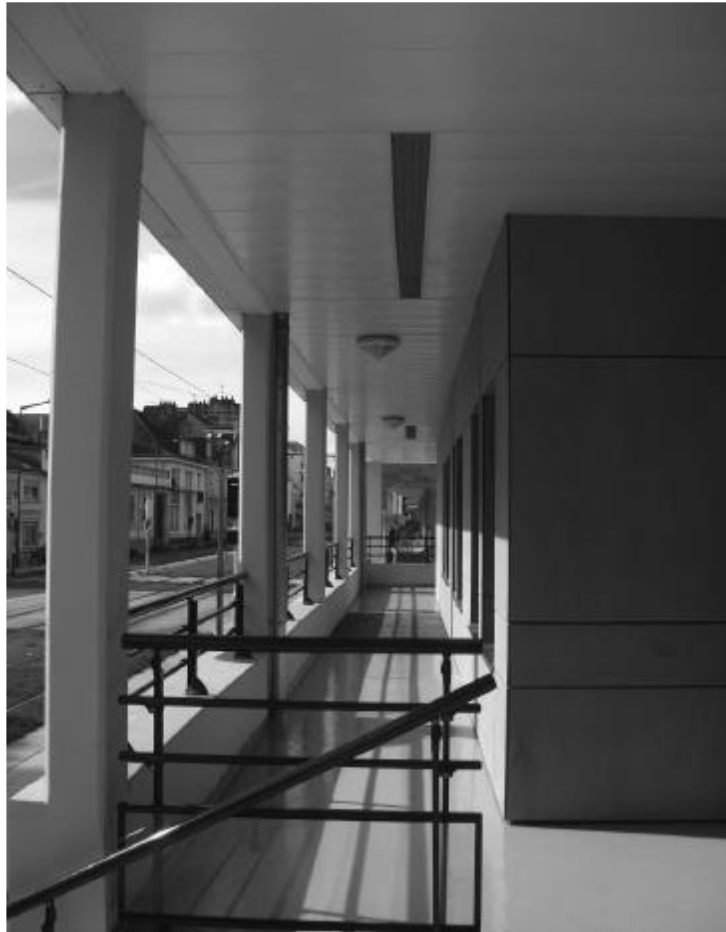
Figure 4 Row of elevated walkways. Access to buildings is difficult, especially for people with reduced mobility. The relation to the street is not direct, which raises multiple problems in terms of urban quality. Source: A. Moreau
