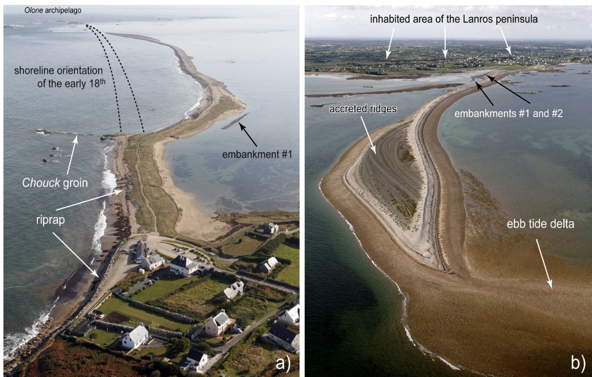
Fig. 3. Aerial photo of the Sillon de Talbert. (a) Photo taken the 23 September 2009 (source: D. Halleux) showing the coastal defense structures on the sandy proximal section; (b) photo taken the 12 September 2007 (source: D. Halleux) showing the tip of the spit with the ridges of accretion and the ebb tide delta.
