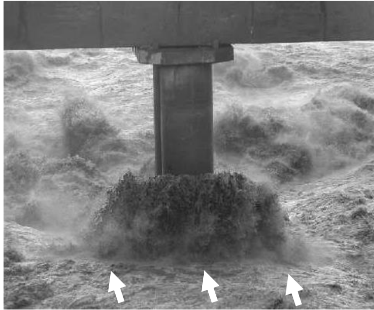
547 Figure 1. Photograph of the wall-jet-like bow-wave around a bridge pier in the "Rivière des 548 Galets", La Réunion Island, France, in March 2006. Courtesy of Paul Bonnet, DEAL 974 (ex 549 DDE 974)
