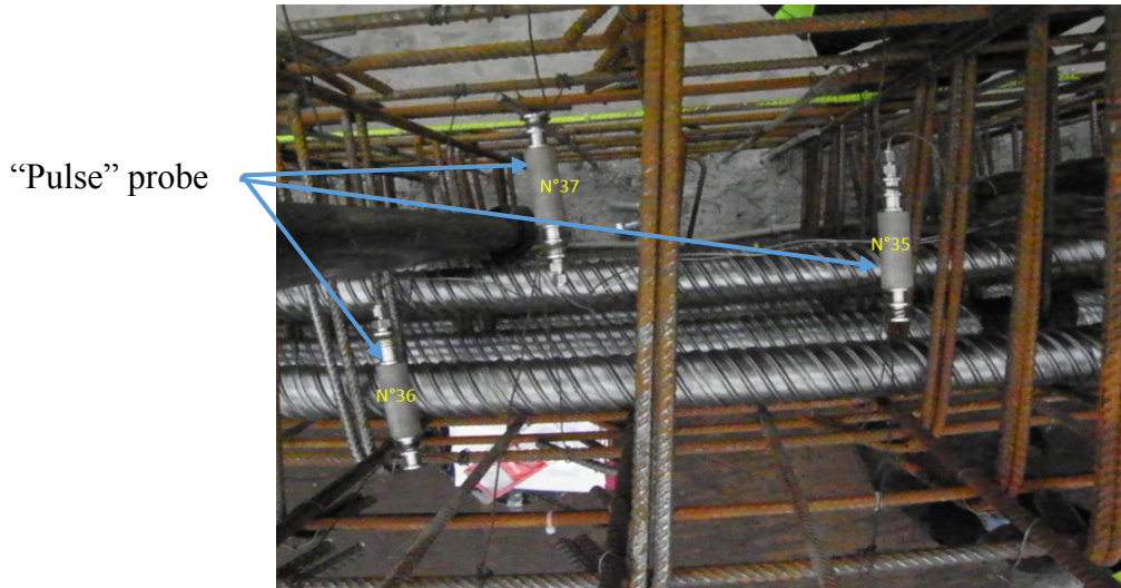
Figure 2. Pulse probes before casting of a reinforced concrete structure.
