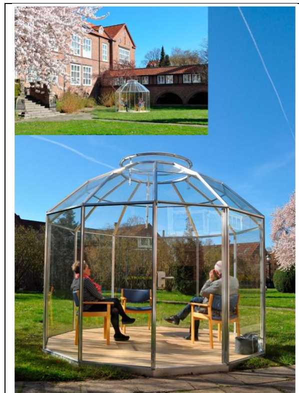
Figure 1: Greenhouse used in Denmark for NDLPDT. This greenhouse is composed with one layer window glass with acrylic at the very top (from Lerche et al).
