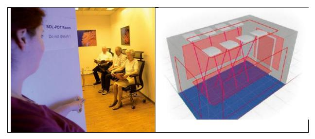
**Figure 8** : SDL-PDT room equiped with this IndoorLux system. Illumination sources are installed at the ceiling of the treatment room.
