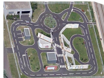
Fig. 23 PAVIN experimental platform (Clermont-Ferrand, France).
