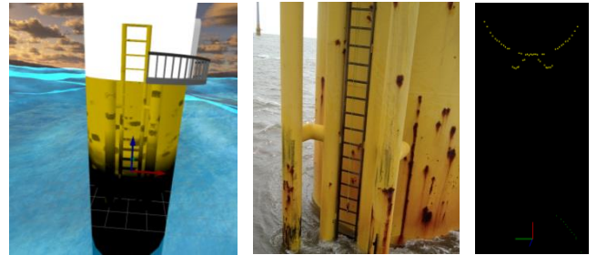
Figure 3 Wind turbine pile - simulated, actual and LIDAR sheet obtained
