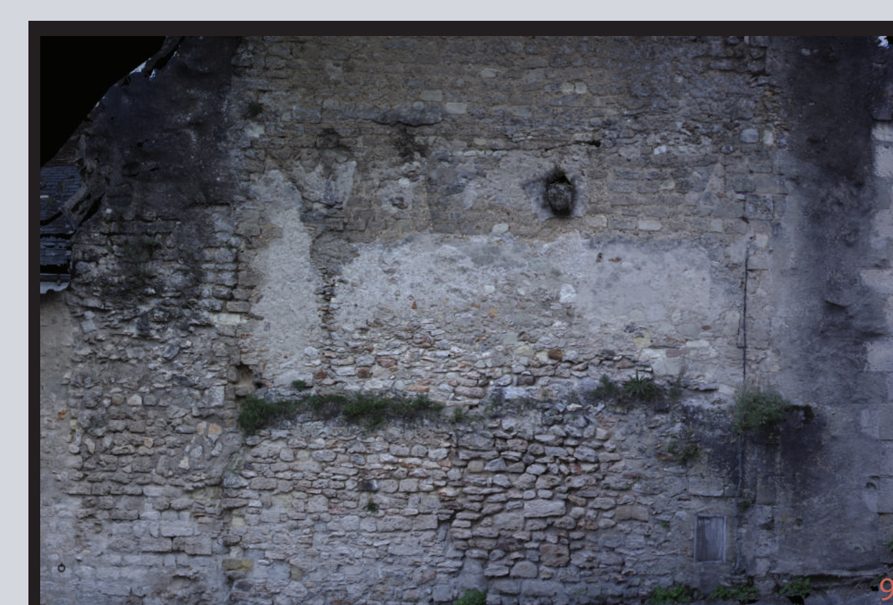
9 - Ortho-image of the west wall of the north transept church.
