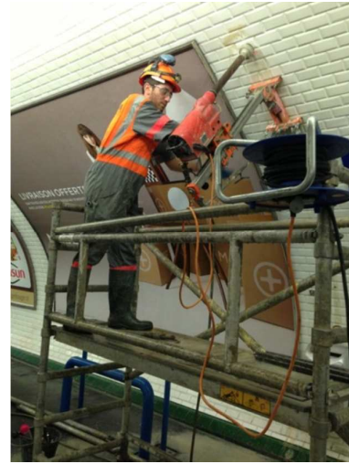
b) Extraction using a 76 mm core drilling sampler
