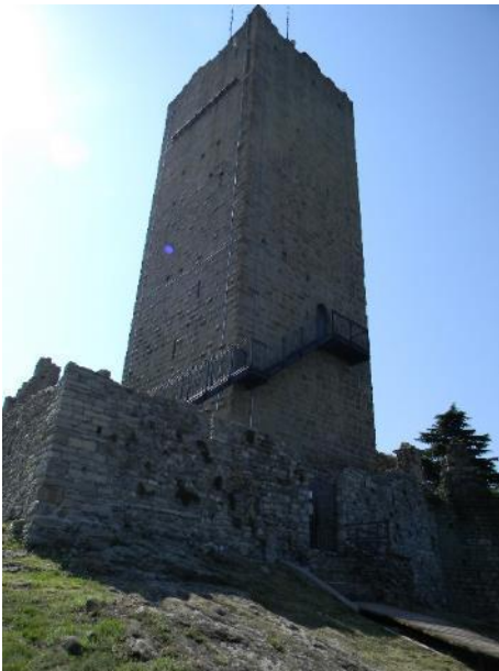
Figure 1 – The Tower of the Baradello Castle, Como, Italy
