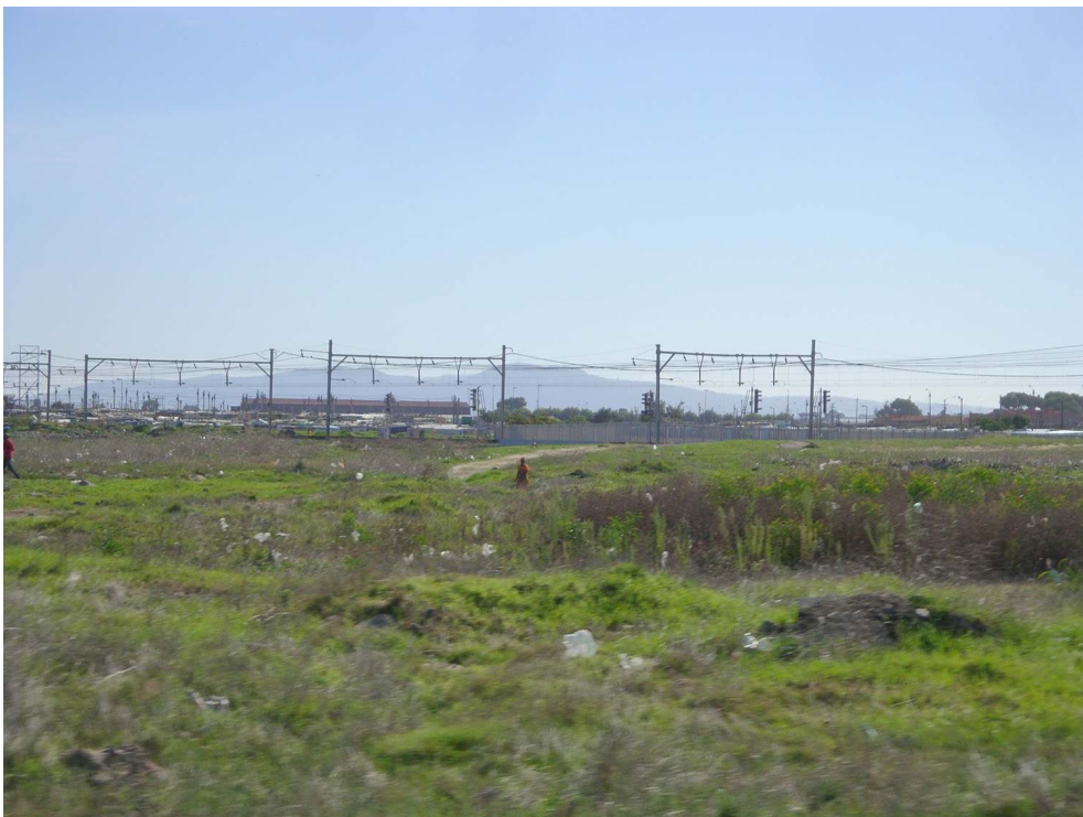
Figure 5: Govan Mbeki Road (formerly Lansdowne Road), Gugulethu.
