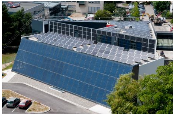
Fig. 1. Global view of the ADREAM Experimental Platform on energy exchanges, LAAS-CNRS Toulouse
