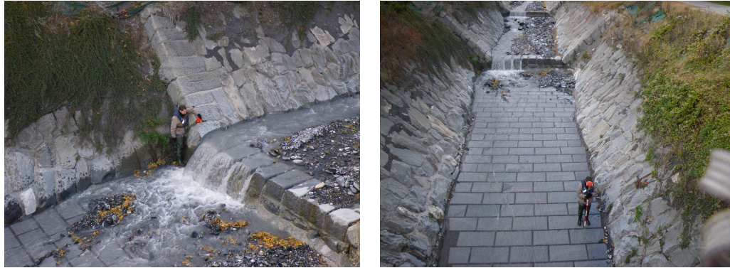
(a) Measuring the cross-section of the main weir (b) Measuring a GRP on the flagstone edges
