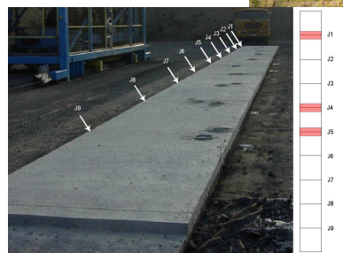
Figure 14 - The white topping specimen
