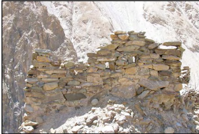
Fig. 40: Multi-colored cobble masonry: stones are mainly cobbles and are of several colors, the most noticeable and characteristic being green. The stones come from fluvio- glacial sediments, visible at various locations in the valley. Tower of Thangring, the wall is about 1 m high. [credits: Devers 2009]
