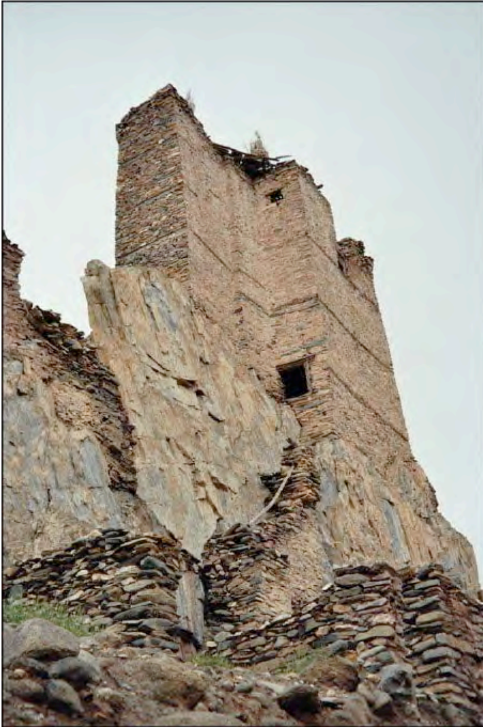
Fig. 38: Hankar: view of the tower from the south-west. Mud- mortared stones with timber lacing. [credits: Vernier 2009]
