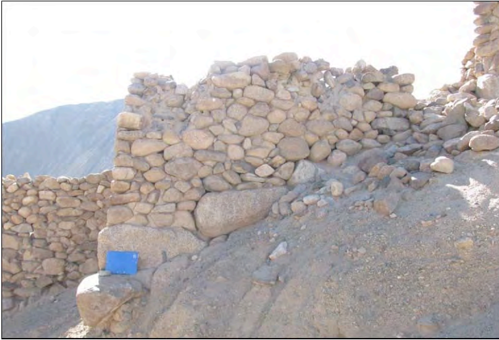
Fig. 46: Masonry of greyish cobbles at the castle of Phey. The blue folder is 24x31 cm. [credits: Devers 2009]
