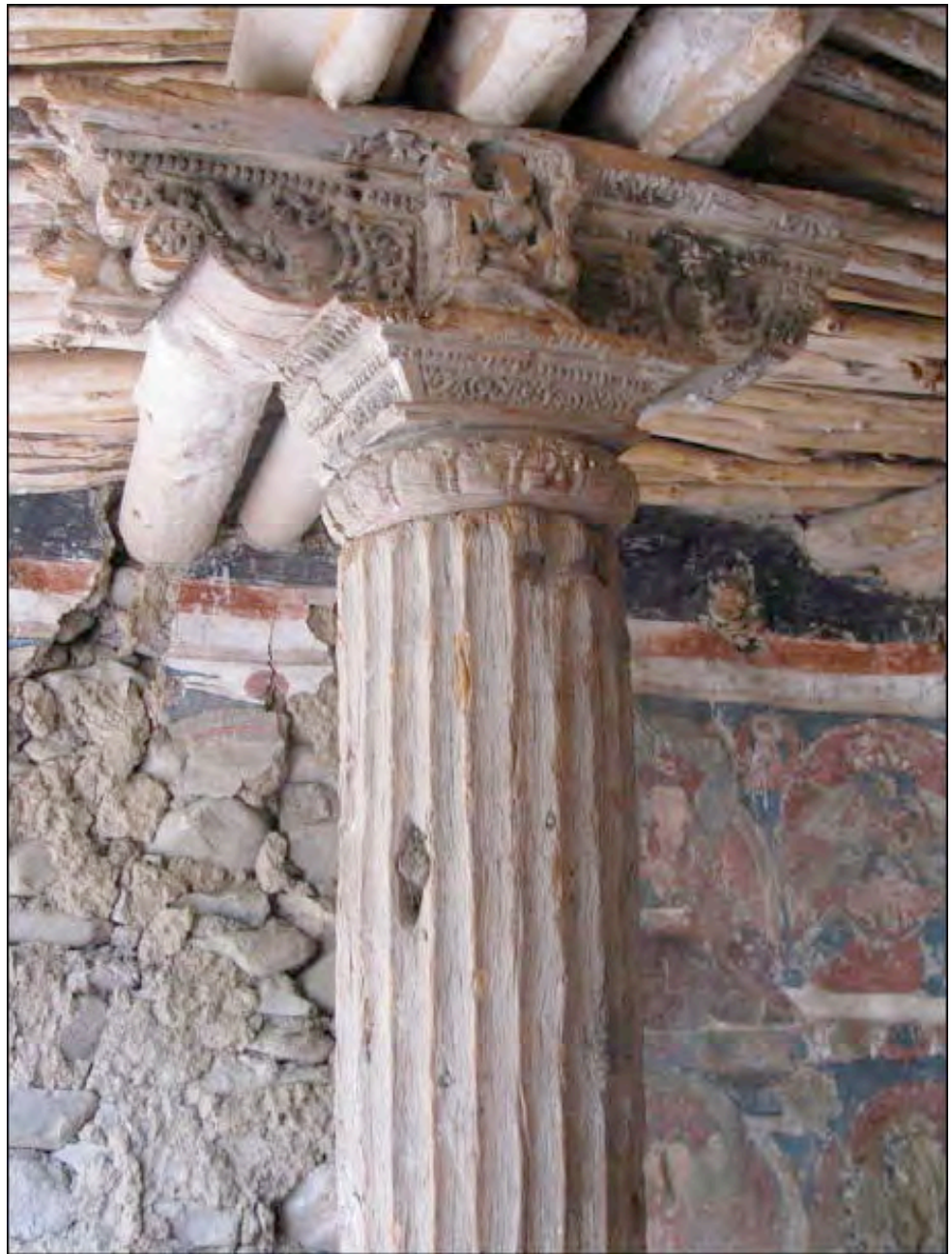
Fig. 26: Markha: eastern side of the fluted pillar and sculpted capital (juniper, 24 cm in diameter, probably 12th century). [credits: Devers 2009]
