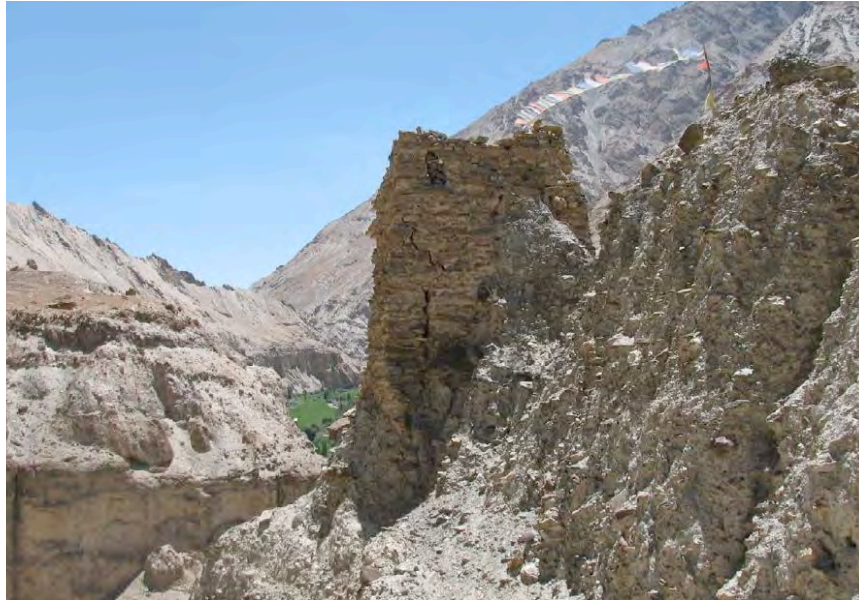
Fig. 3: Kaya: tower of the castle viewed from the west (mud-mortared stones, r. 3x3 m). [credits: Devers 2009]
