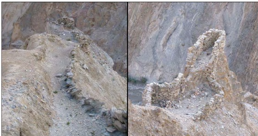
Fig. 34: Teacha: West crag: the allure on the top of the crag, with the tower A on the background viewed from the north-eastern end of the allure [left]; one of the defensive structure (B) viewed from the south-east [right] (dry stone masonry, walls are r. 80 cm high and 6 m long). [credits: Devers 2009]
