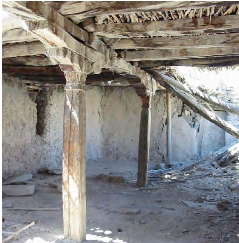
Fig. 23: Markha: "reception hall" of the second floor, with timbers of square section. [credits: Vernier 2004]
