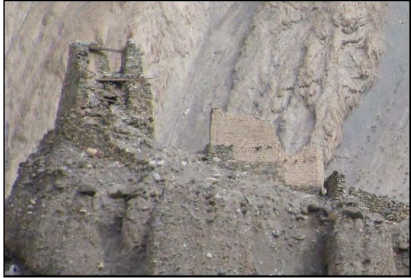
Fig. 22: Markha: tower of the northern crag (left, mud-mortared stones) and possible grainhouse (right, mudbricks: 40x20x10 cm) viewed from the west. [credits: Devers 2009]
