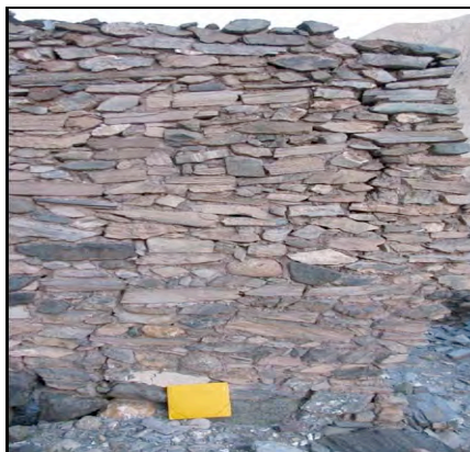
Fig. 44: Masonry with a predominance of schist. This wall is one of those made with red mortar at Hankar. [credits: Devers 2009]
