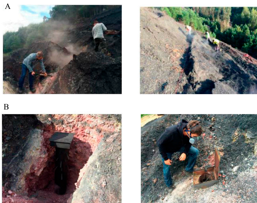
Figure 9. (A) View of the field installation of the fiber optic temperature cable; (B) one of the structures where the gas sensors/point temperature sensors were installed.
