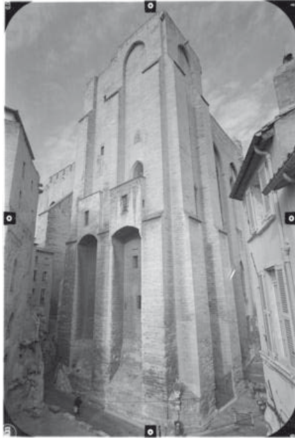
Tour Saint-Laurent south-east overview
