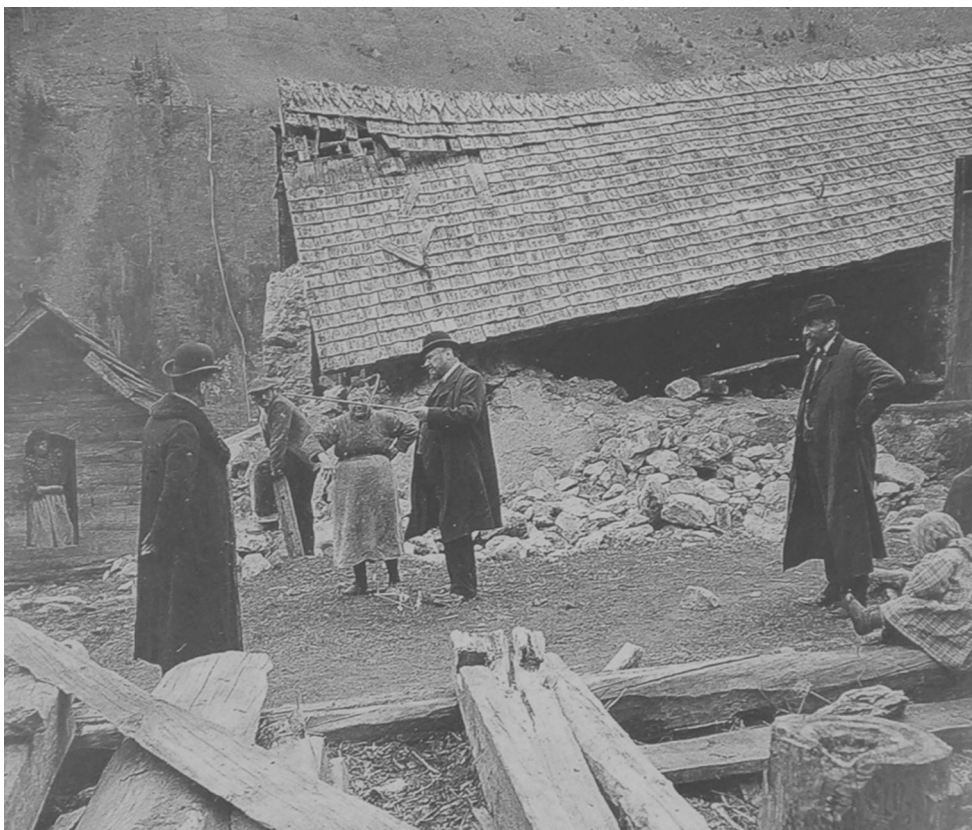
Fig. 4 April 29, 1905 earthquake: partial collapse of a house in La Joux near Argentière (coll. Jules et Michel Payot; Cuenot 2015). For location see A5 in Fig. 3
