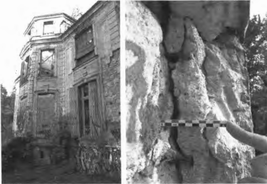
Figure 6: Goussainville, nineteenth century house. Left: general view. Right: detail on the layers of the rendering. (Tiffanie Le Dantec, 2015)
