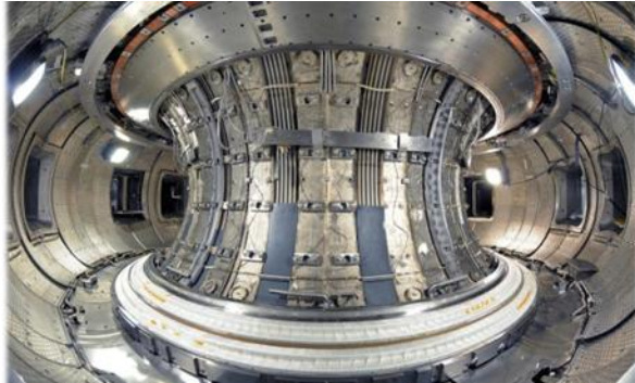
Fig. 2. Inside the vacuum vessel in June 2016. Lower coil winding is still visible.
