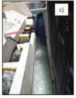
**Figure 1:** a) The view of submerged studied low-sloping rack with two entrances, b) bypass immediately after the entrances, c) the following bypass channel and the fishpass (left side of the photo) of the Auterrive HEP.
