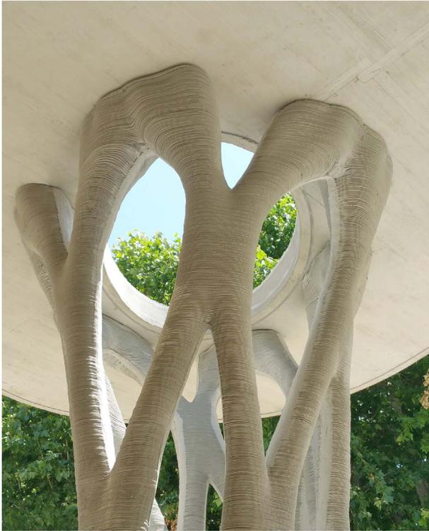
Fig. 4. Printed pillar in Aix-en-Provence (XtreeE, 2016).
