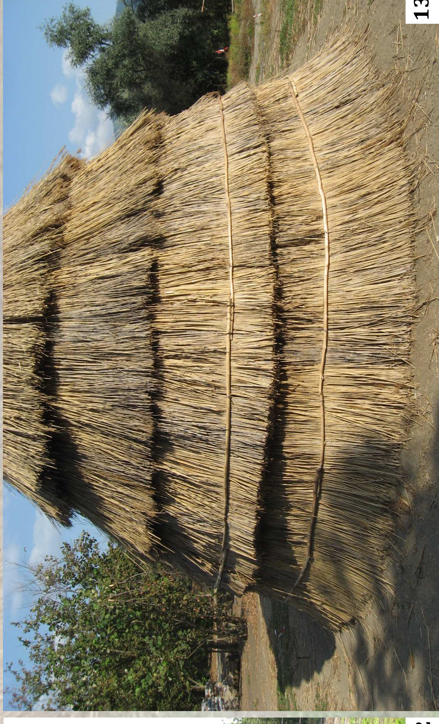
9 Making of the roof-wall in hut 4 replica (Park of San Paolo Belsito)
