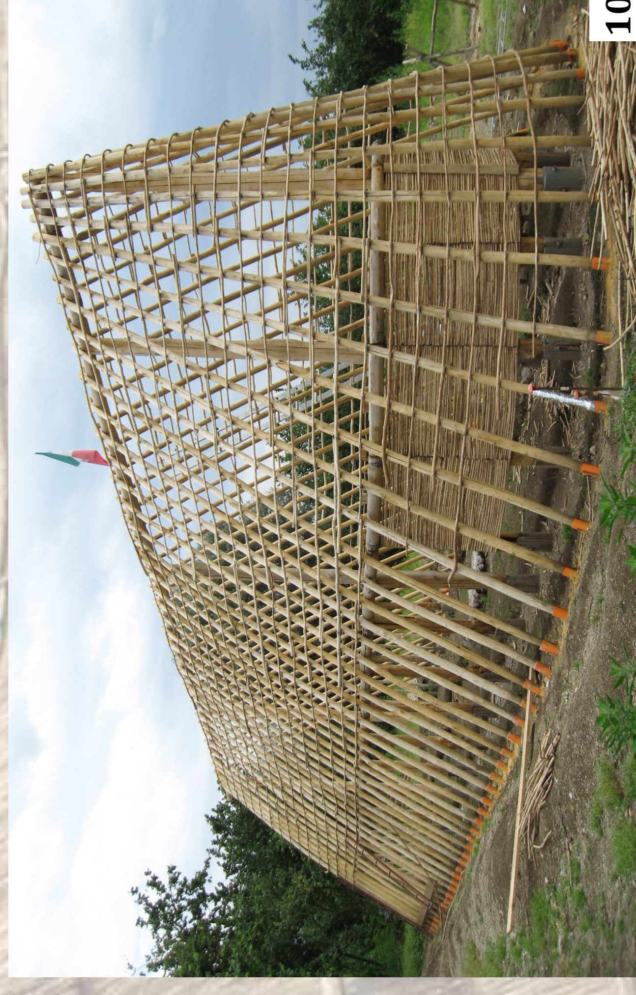
9 Making of the roof-wall in hut 4 replica (Park of San Paolo Belsito)
