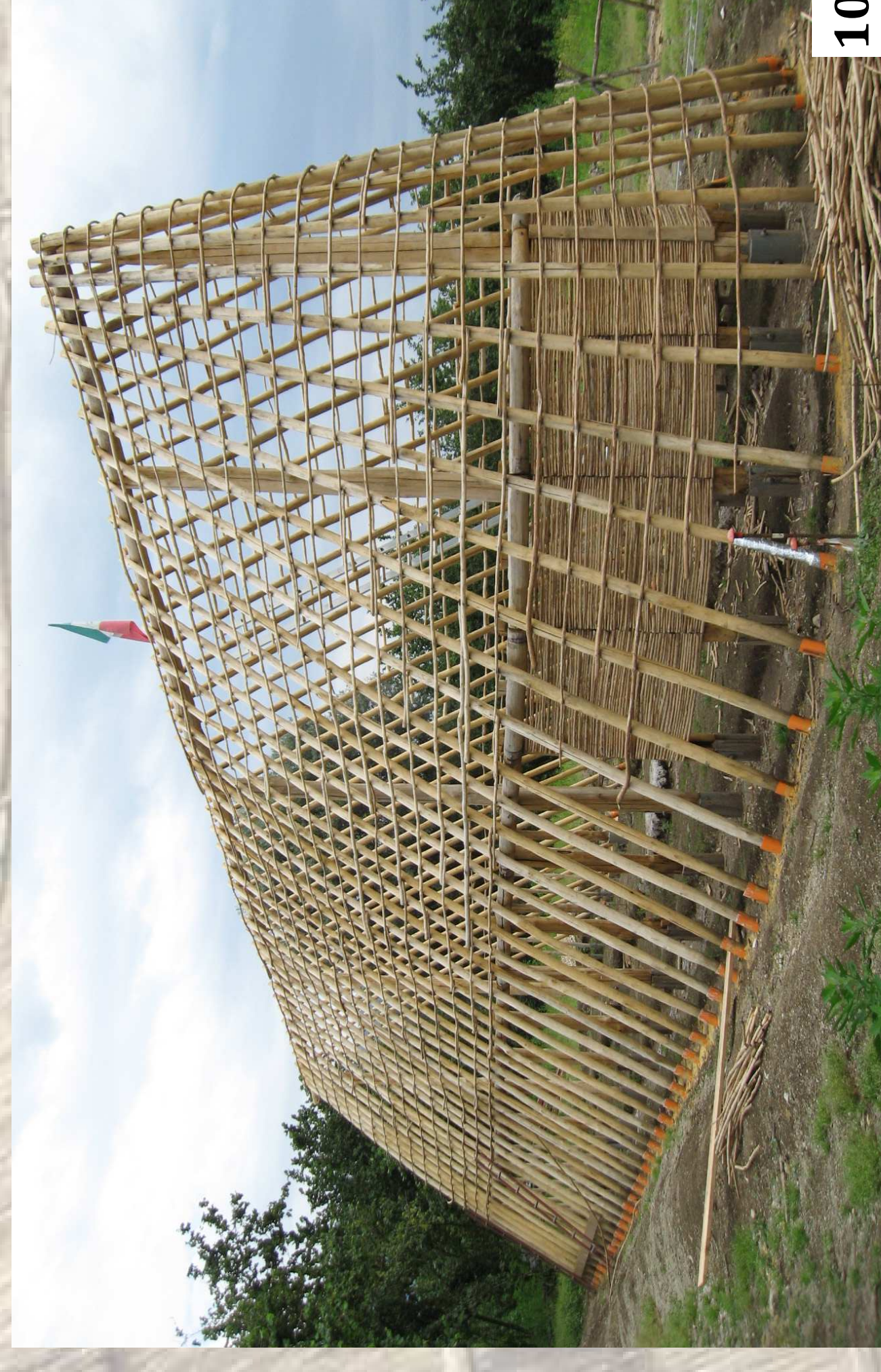
10 Making of the roof-wall in hut 4 replica (Park of San Paolo Belsito)
