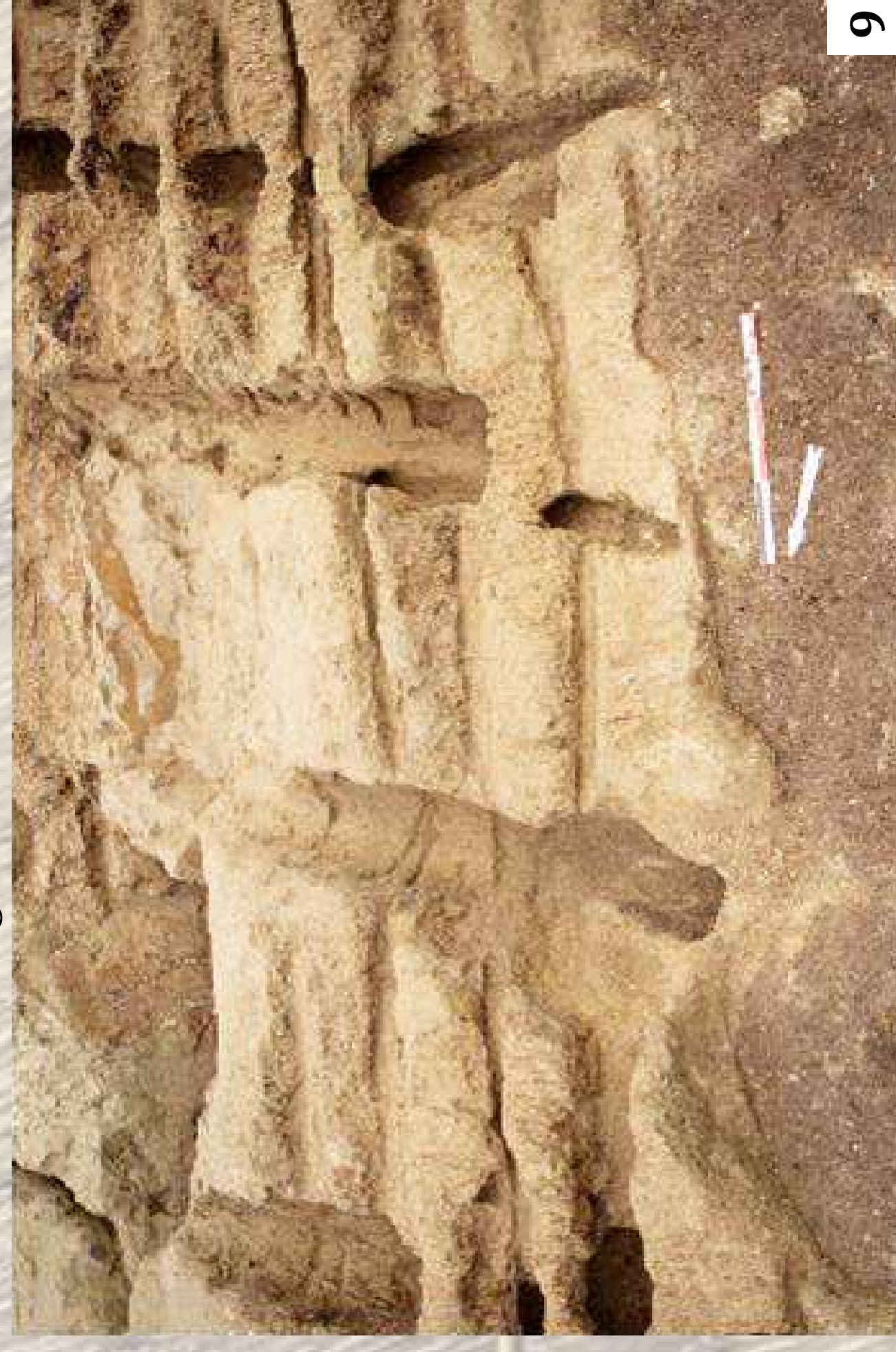
5 Building detail of infill-walls anchoring
