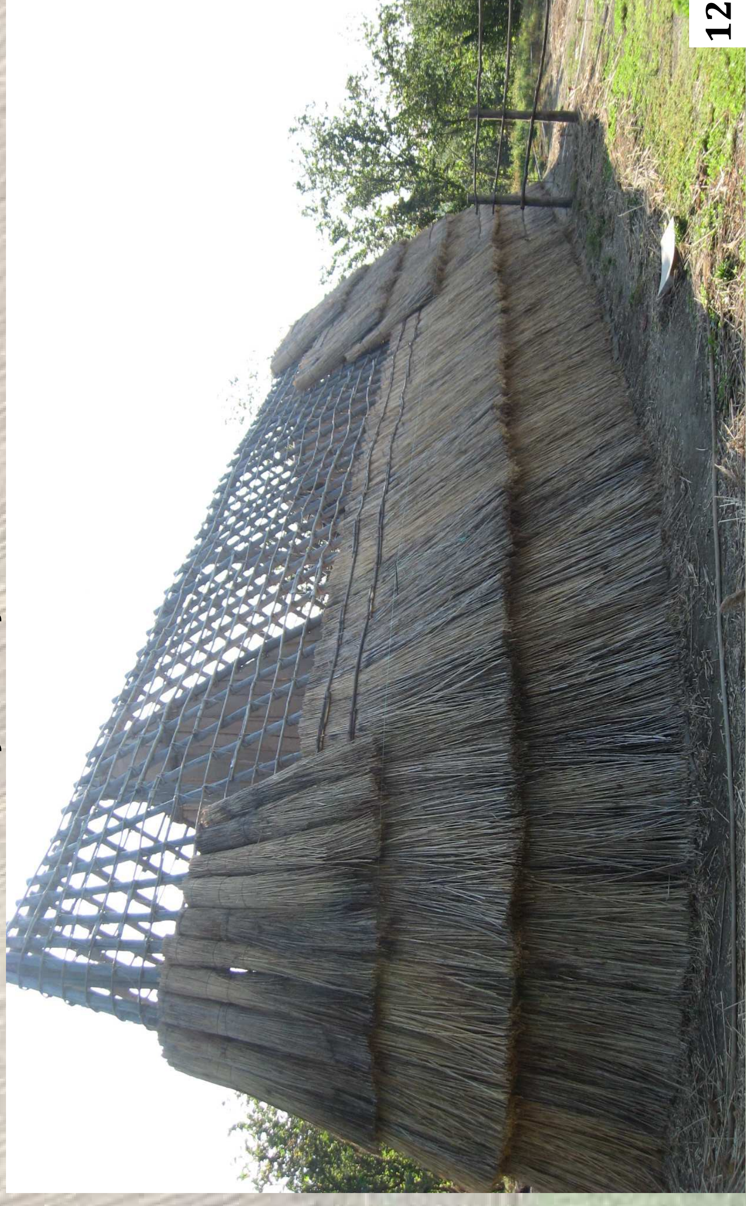
9 Natural cast of the reclined poles and of the horizontal battens of the roof-wall
