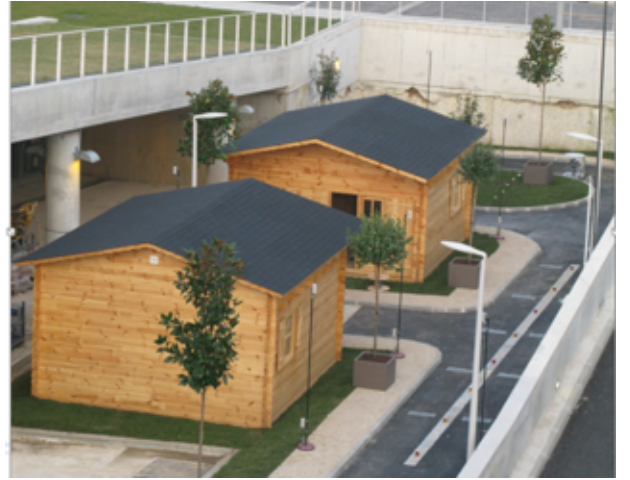
Figure 3: Chalets of the “Sense-City” equipment located at IFSTTAR Marne-la-Valle, France
