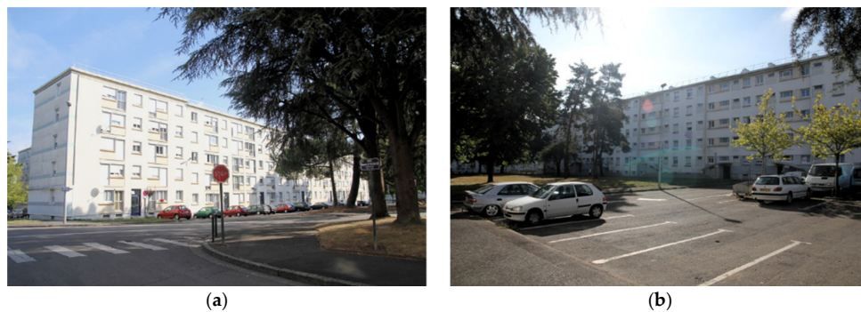
Figure 2. The Dunant building: (a) southern facade; and (b) northern facade.
