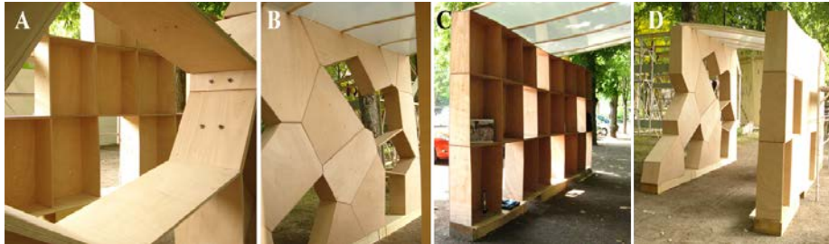
Figure 8. Finished wall prototypes. A, Grid-pattern wall view through a voronoi cell. B, Voronoi-patterned wall. C, Grid-pattern finished wall. D, Finished prototypes.
