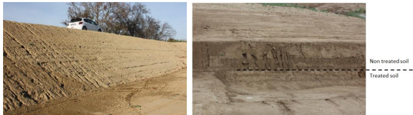
Figure 5. Left : Non treated soil (Zone I) at left hand side, with erosion channels ; lime treated soil (Zone II) at right hand side, with no erosion channel.
