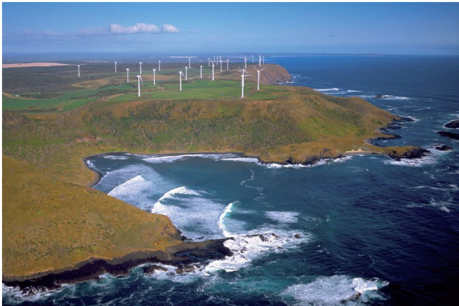
Figure 3.4: The Woolnorth wind farm at a cliff.
