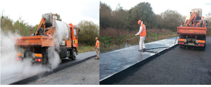
Figure 4. Application of tack coat.
