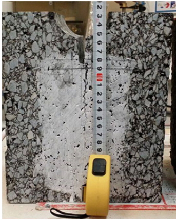
Figure 9. Determination of the depth of the crack using whitening chalk powder.
