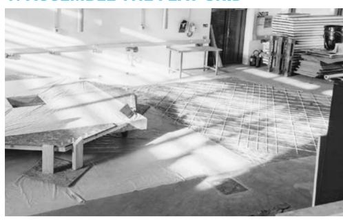
Prepare the glass fiber reinforced rods for the gridshell: cut the rods at the required length and drill the holes that will receive the connectors at a constant step-size. Assemble the flat grid on the ground. This is unskilled work that consists in bolting together the rods at each node.
