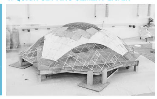
Prepare the formwork with a quick-setting cement layer. This intends at reinforcing the fabric in form in order to prevent the sagging between the rods. Because in our prototype this layer is visible on the underside, a large amount of time was spent in the finishing and smoothing.
