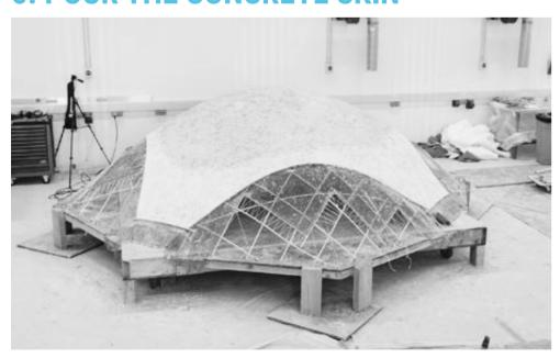
Pour the concrete. The concrete was prepared and poured in three batches of 50 I each, for a total mass of concrete on the structure of 348 kg, and average thickness of 15.4 mm.
