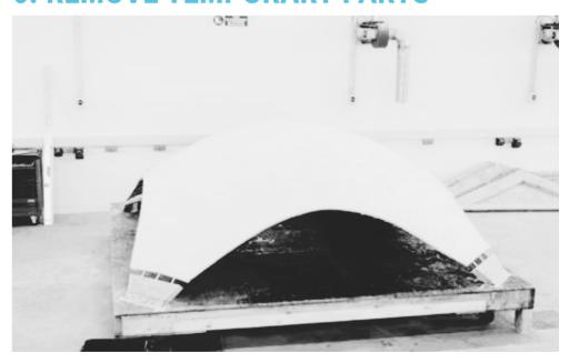
Cut away the temporary parts of the gridshell after the concrete cured seven days. Protect the concrete skin with lime whitewash.
