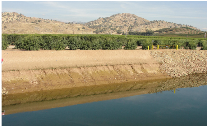
Figure 1: Lime-treated section of the Friant-Kern Canal (taken in November 2010) on the left part; the right part consist of original, untreated slope covered with gravel.
