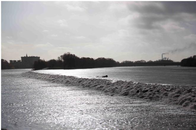
FIGURE 6 : DEVERSOIR LATERAL DU CANAL DE FUITE DE L'AMENAGEMENT DE LA CHUTE DE VALLABREGUES
