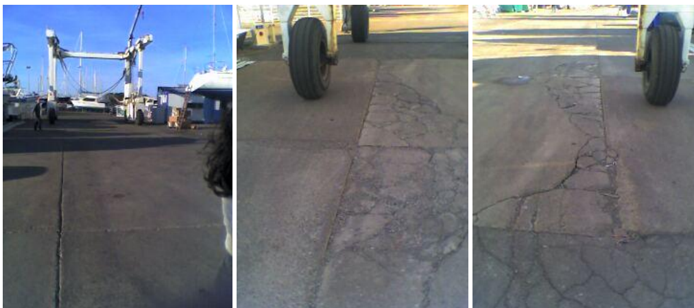
A: concrete slabs and the “Port Olona” Travelift
