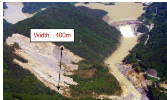
Fig. 3. Large landslide downstream of the Tsukabaru dam.
