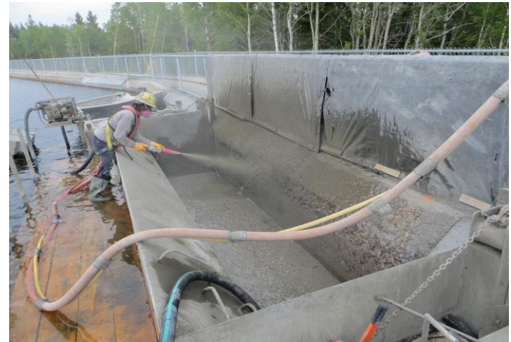
McCormick Dam and Power Station, QC, CA – KING Shotcrete Solution
