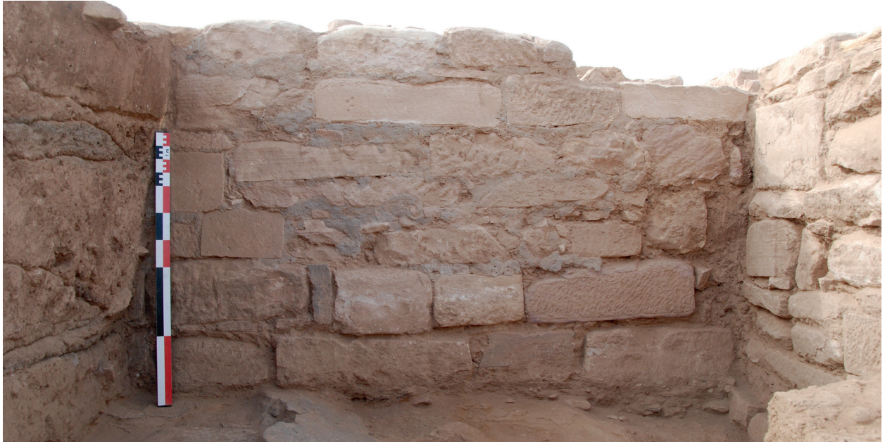
Fig. 13. North facing of wall 60804.
