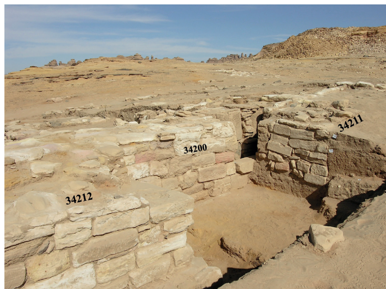
Fig. 14. Trench B. Gate 34234 in the center-right, buttress 34211 to the right, rampart 34200 in the center and tower 34212 on the left. The blocking 34238 and the upper threshold visible in the gateway. View from the south-west.
