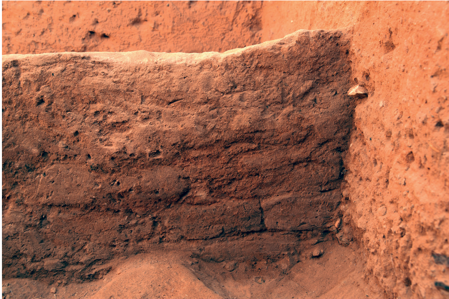
Fig. 8. West facing of mudbrick wall 35201, southern end, looking north-east.
