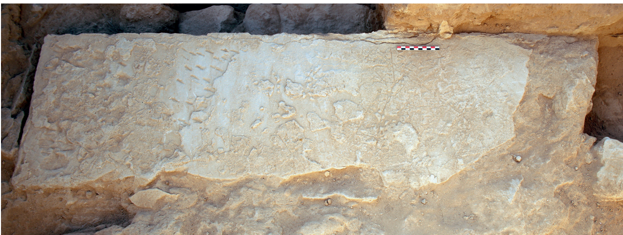
Fig. 10. Block from wall 35049 showing trace of a vertical joint, viewed from the north-west.
