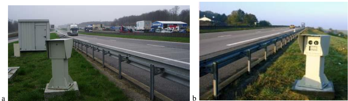
Fig. 1. Standard WIM station in France: (a) WIM sensors in the pavement; (b) cameras in the road side cabinet.
