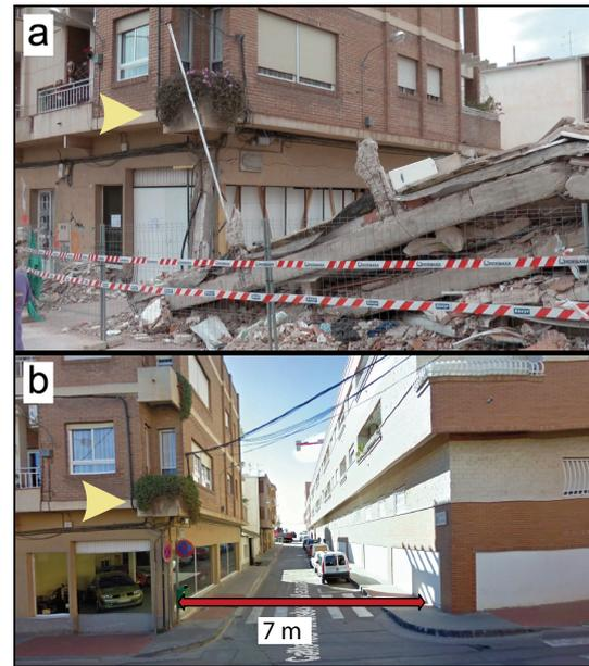
**Figure 5.** An example of how maximum impact distance was evaluated. Photographs: (a) Marc Bertran Rojo and (b) Google Street.
