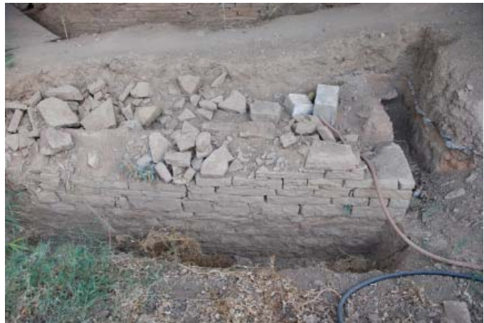
Fig. 14. Ancient stone wall exposed during illegal excavations in Sector C
