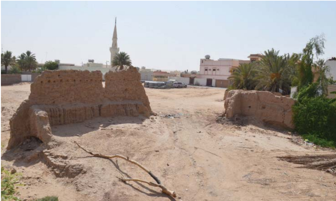
Fig. 20. The southern and western walls, looking south
