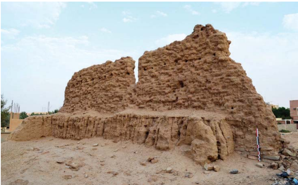
Fig. 19. The “interior” face of the southern wall, looking south
