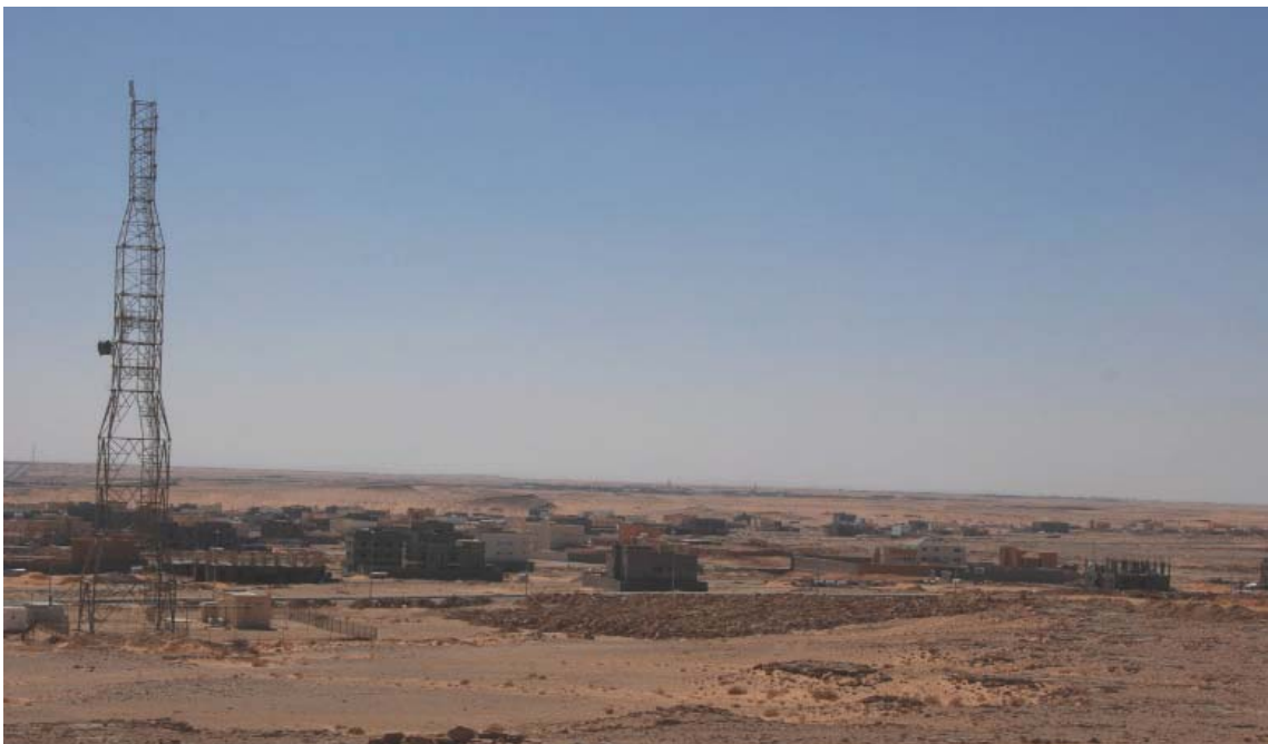
Fig. 6. Residential quarter extending on the plateau, located south of Sector C
