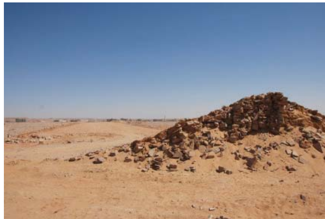
Fig. 8. The segment of the enclosure wall (unit 4) cut in 2011, near the road in progress
