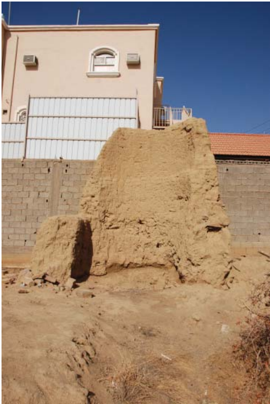
Fig. 3. Mud-brick tower in Dūmat al-Jandal endangered by modern construction
