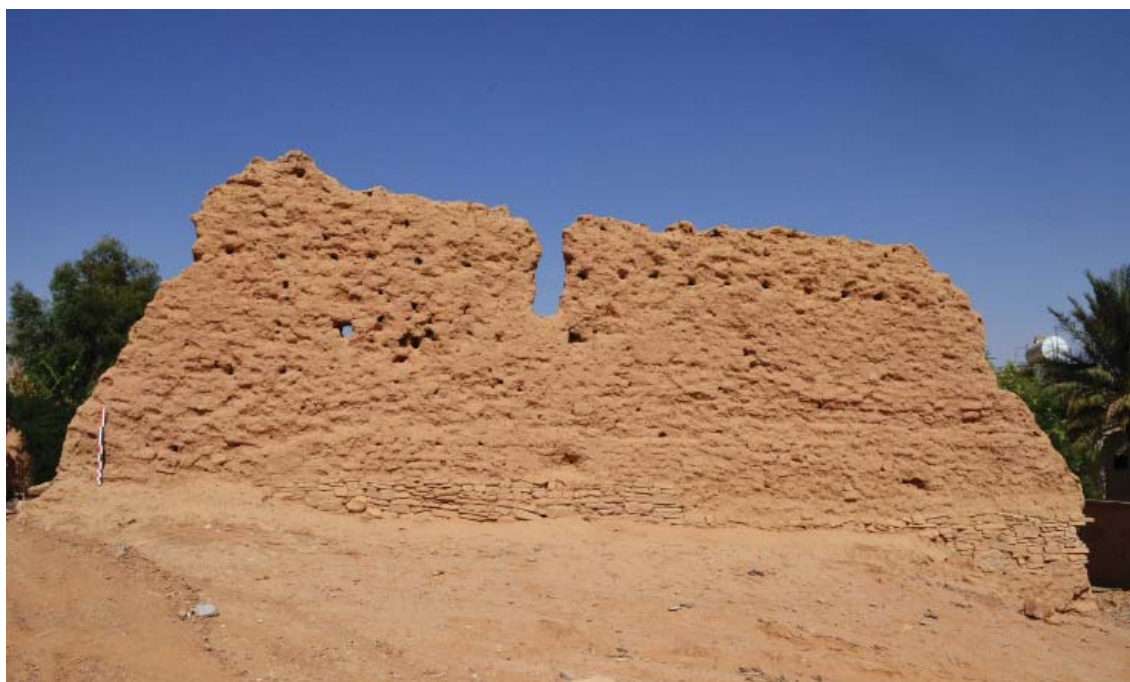
Fig. 18. The “exterior” face of the southern wall, looking north
