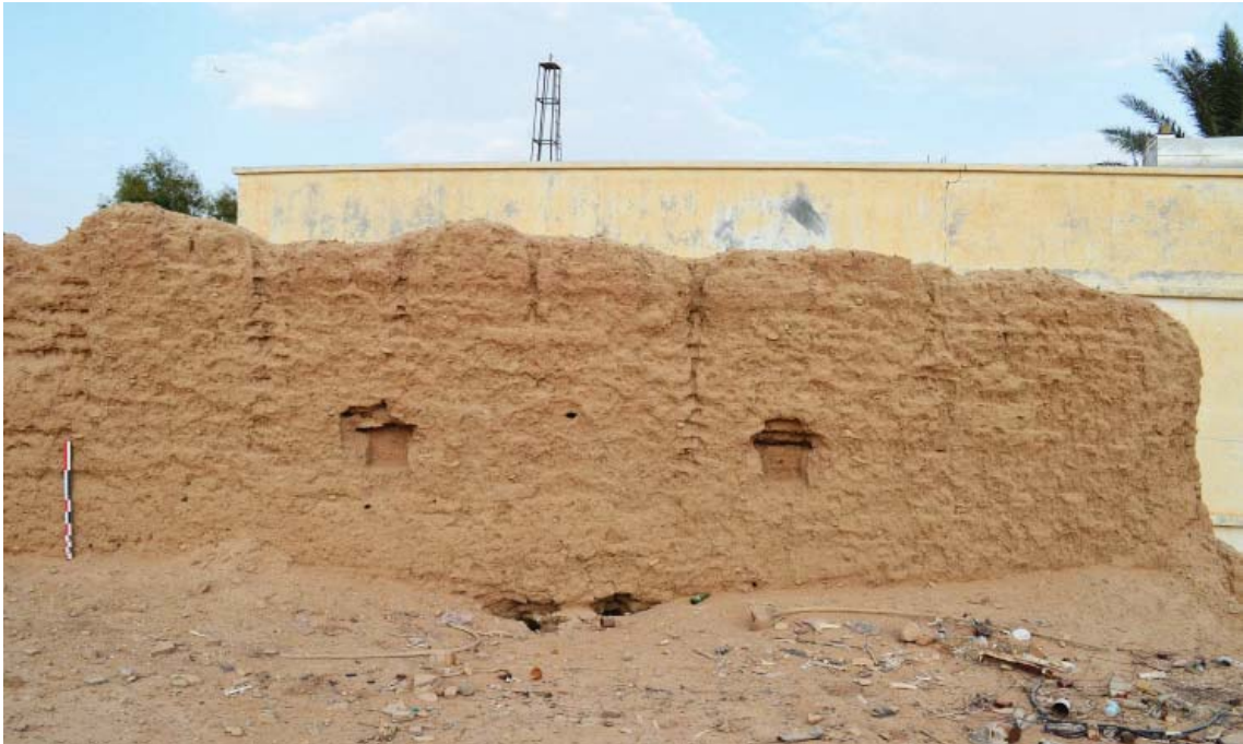
Fig. 22. The “interior” face of the eastern wall, looking east
