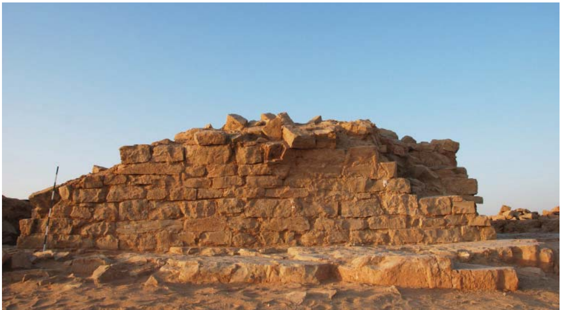
Fig. 39. Wall M2024, looking south
