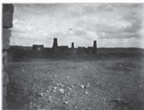
Fig. 9. The Qasr Jawhar in 1900 (Forder 1905: 204), probably looking south-east
