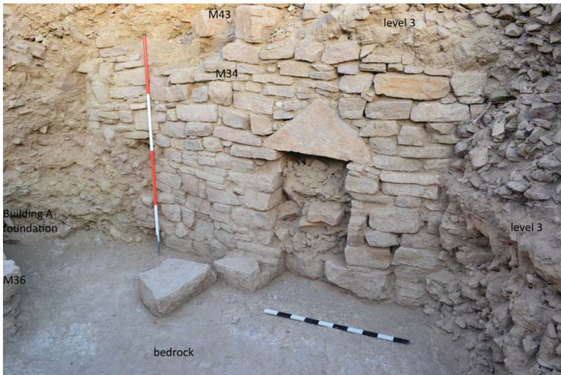
Fig. 47. M34, built directly above the bedrock and covered by Level 3. View from south-east
