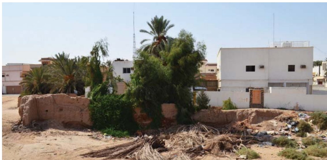
Fig. 17. The “interior face” of the western wall, looking west
