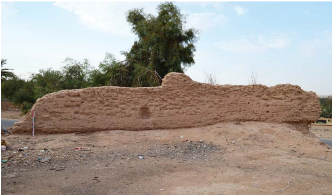
Fig. 23. The “interior” face of the northern wall, looking north
