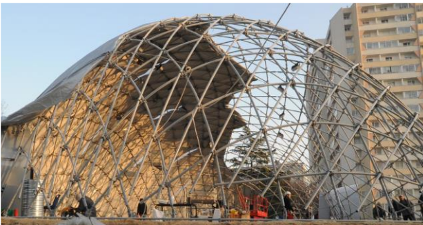
Figure 2: Crêteil gridshell, covering in progress.
