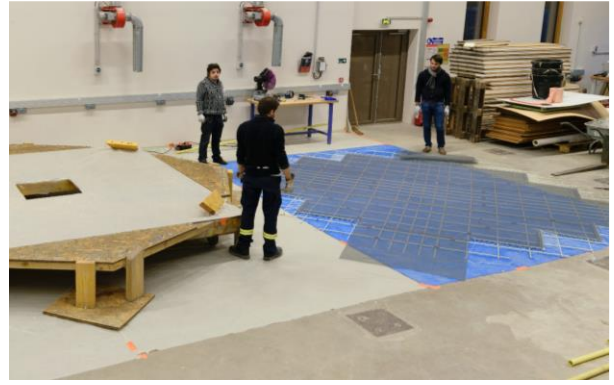
2. Mesh formwork preparation
