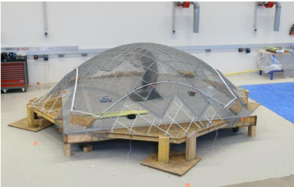
3. Gridshell erection and bracing
