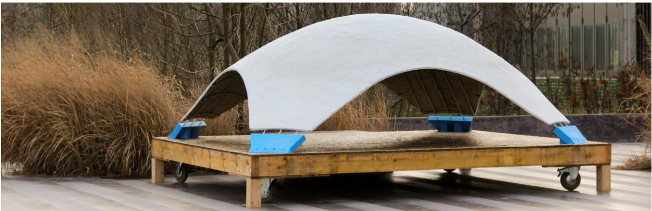
Figure 1: 3-by-3-meters prototype of GFRP gridshell braced by a concrete envelope built at the Ecole des Ponts ParisTech.
