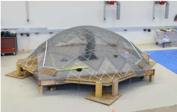
3. Gridshell erection and bracing
