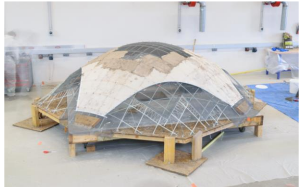
4. Quick-setting cement placing
