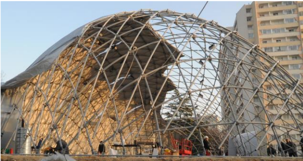
Figure 2: Créteil gridshell, covering in progress.
