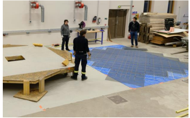
2. Mesh formwork preparation
