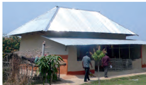
From the top: improved existing house in Chittagong; Safer house models in Dinajpur and Rajshahi
