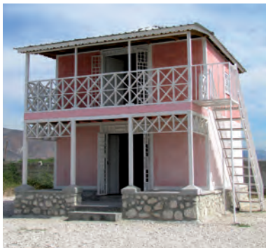
Haiti: traditional timber frame construction in urban area, 2-storey housing for dense area, bus station
