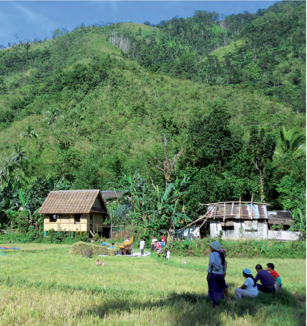
Philippines: existing house (right) and houses rebuilt after 2013 typhoon Haiyan with improved local techniques and materials (left)
