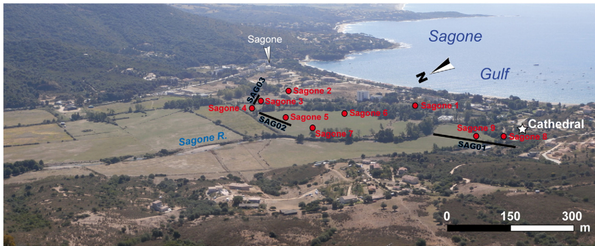
Fig. 5. Oblique view of the Sagone coastal/deltaic plain with location of the boreholes drilled (red circles) and the ERT profiles (black lines) established for the present study.
