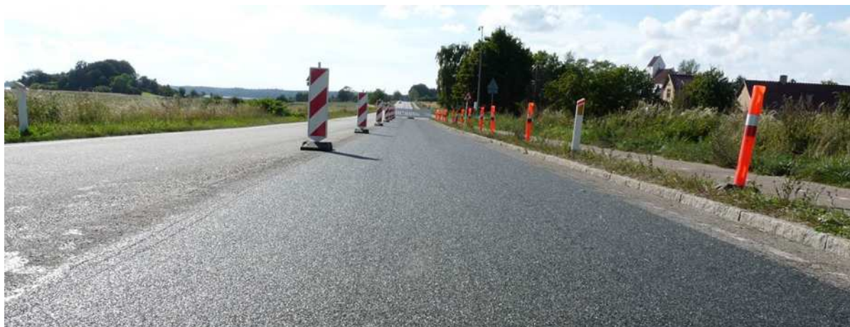
Figure 1 - The PERS test section just after construction.
