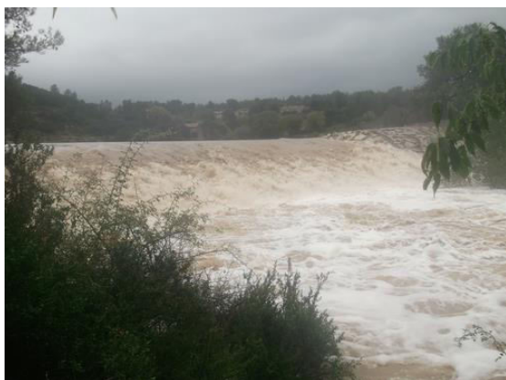
Figure 7. The Roquemaillère basin safety spillway, October 10, 2014, at 9:30, shortly before the flood peak (estimated Q = 68m 3 /s).
